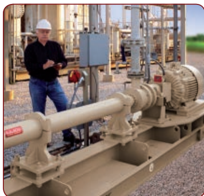
Long view: these multistage pumps can replace other high-pressure types
