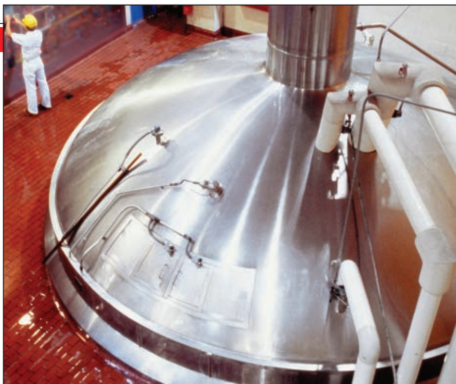
FIGURE 1. Many batch automation vendors are enabling batch functionality at the controller level
